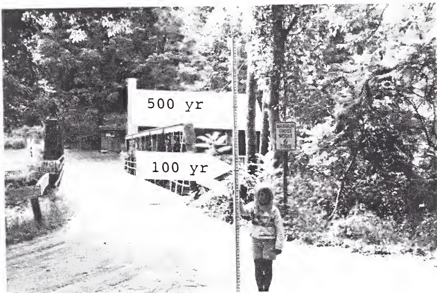
Figure 2. West side of Foundry Road bridge.
